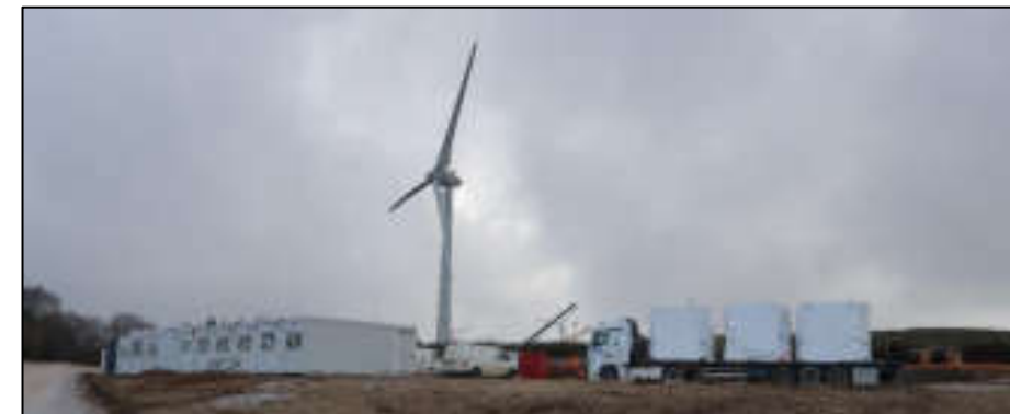
Base vie Source : Artifex 2018
